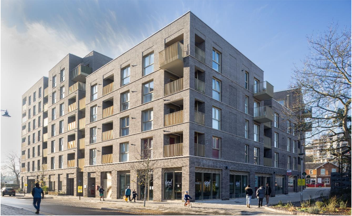
BLOCK D – TRINITY PLACE, YORK ROAD
